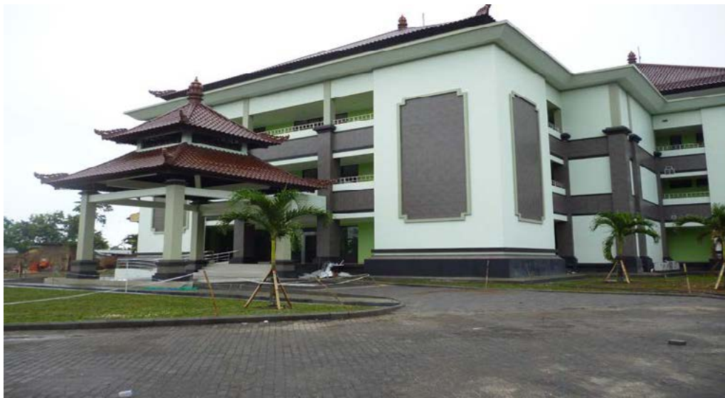
Pc. 1 Treatment Building seen from East
