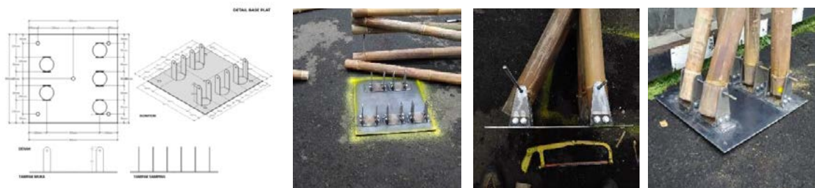
Figure 8 steel plate: the connector between bamboo and foundation
