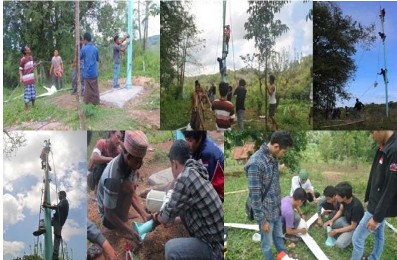
Figure 11 Construction of wind turbine which has been done by IbM team together with the local community of Rembitan village.
