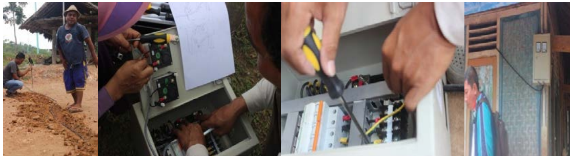
Figure 13 Installation of electrical panel on a house of local community.
