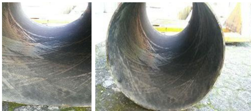
Figure 1. Internal Condition of FRP Pipe Sample
