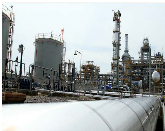
Figure 9 Picture of Surface Production Facilities
