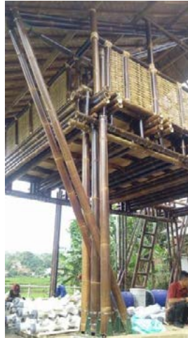
Figure 7 interlocking multi-layers bamboo system
