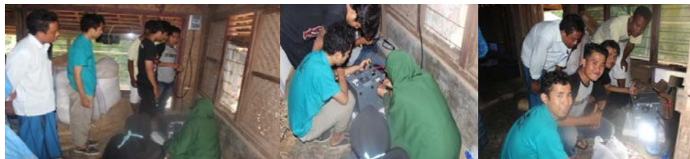
Figure 14 Installation of additional equipment, and the bulb light is shining.
