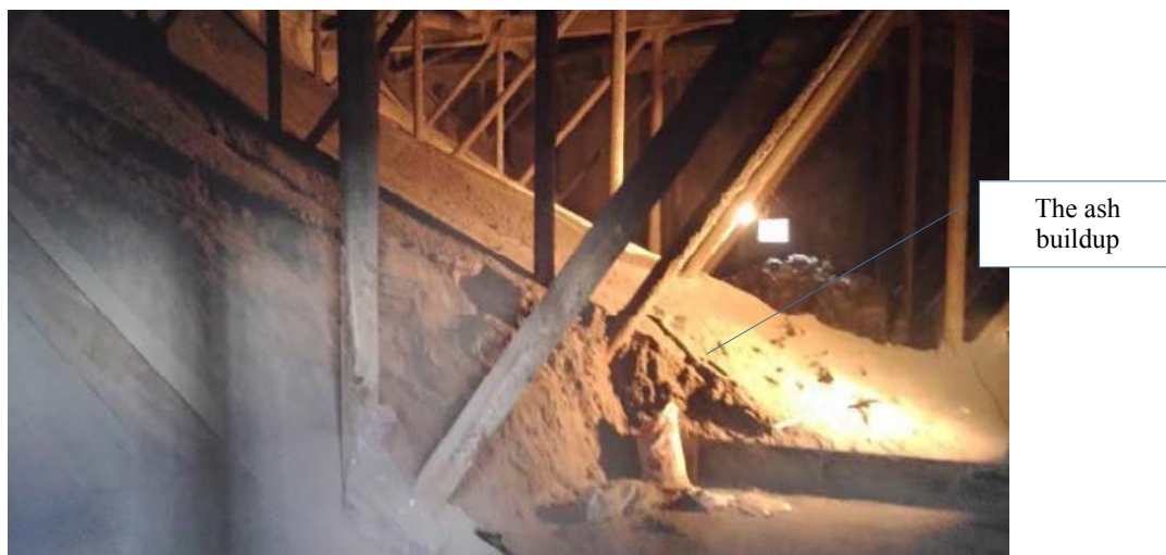
Figure 11. Ash buildup in economizer bottom area.
