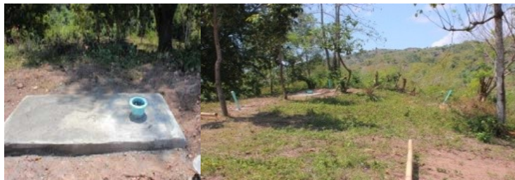
Figure 9 Turbine foundation which has been constructed perfectly by the local community.
