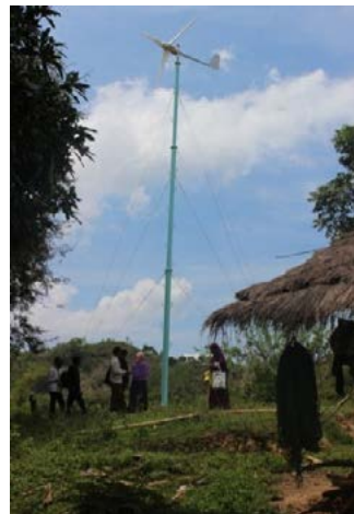
Figure 12 Results of wind turbine construction.
