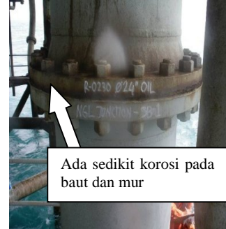
Gambar 17 Tampak dekat flange Line B [8]
