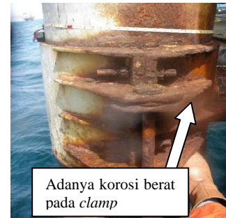
Gambar 18 Tampak dekat clamp Line B [8]
