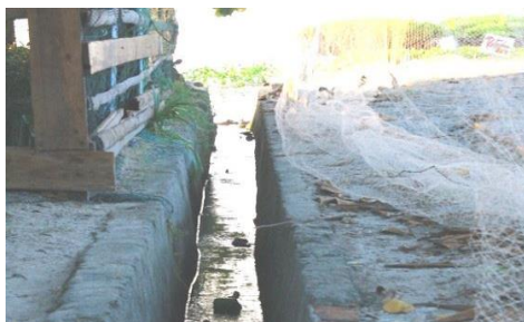
Fig 4. Drainage system in Pramuka island, the surface runoff directly to the sea 36
