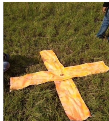
Figure 4. Installation of Premark
