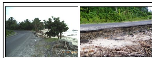
Figure 1. The condition of the west cross road in Lemong Sub-district has been affected by abrasion
