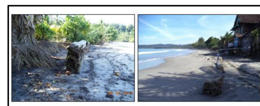
Figure 3. The condition of the coast behind Balam Village
