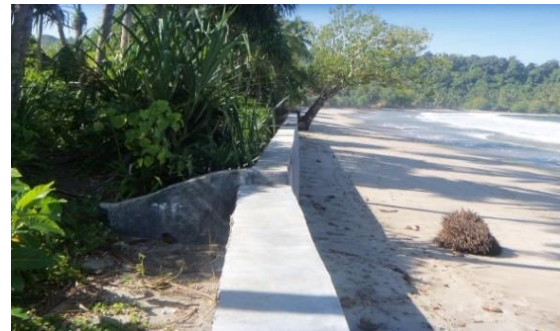
Figure 14. Condition of the coast in 2020 at Balam Village, at first it was a village road
