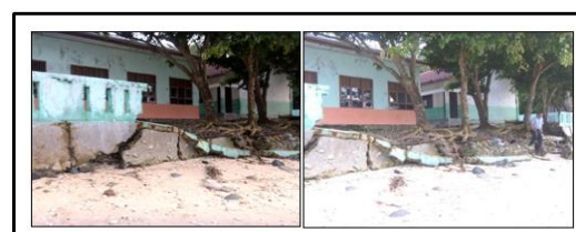
Figure 2. The condition of the coast behind SMAN 1 Lemong
