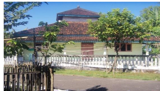
Figure 15. The condition of the village road was moved about 50 m from the beach
