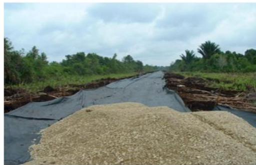
Figure 12: Application of Woven Geotextiles (woven)
