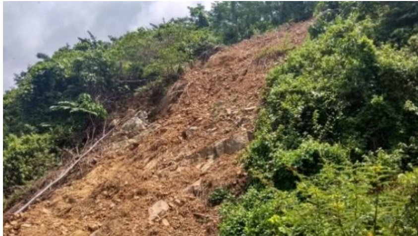
Fig. 10. Landslide Prone Areas (a and b) in Pekon Tanjung Siom Coordinates: 5°33'54" South Latitude 104°44'45" East Longitude
