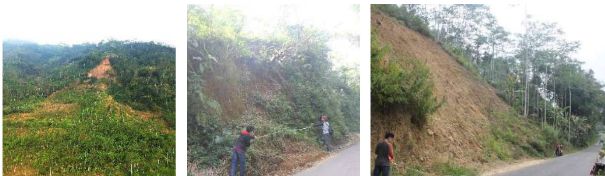
Figure 4. Landslides in Karangkoobar Catchment
