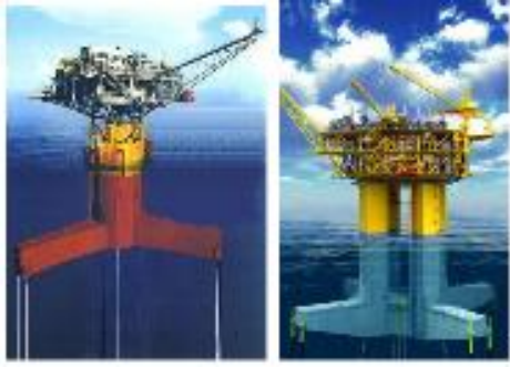
Gambar 1 Contoh Tension Leg Platform https://www.rigzone.com/training/insight.asp?insight_id=305 , 28 Maret 2022
