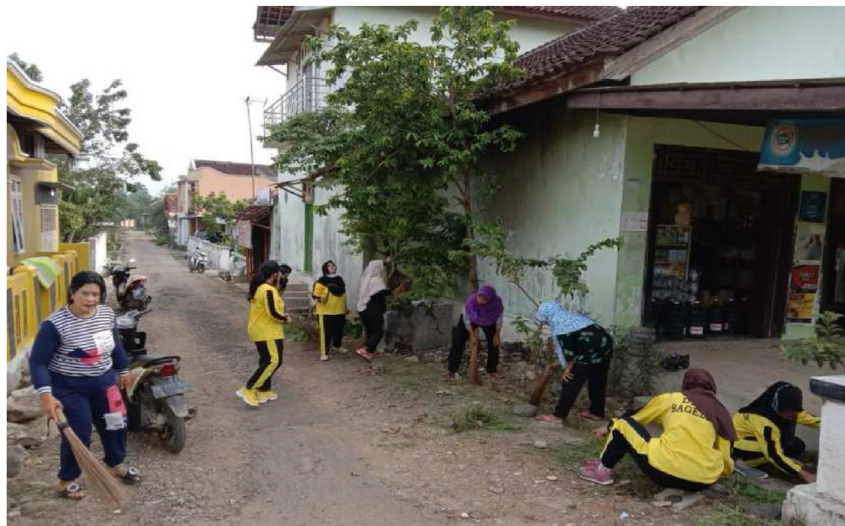
Figure 6. Clean the drainage's activity.
