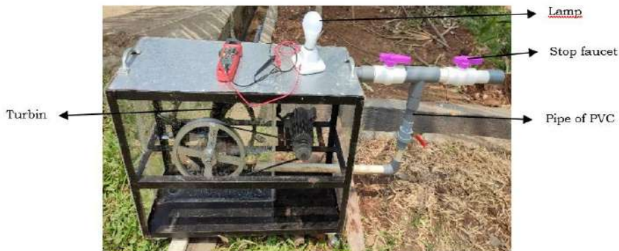
Figure 4. Suite tool installed.
