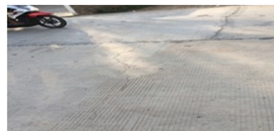
Fig. 3. Single crack lying a cross the rigid pavement with fine cracks
