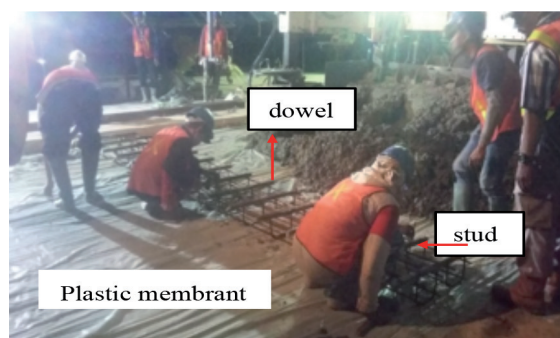
Figure 8. Dowel baskets placed on an LC. Red line: Dowel. LC: Lean concrete.
