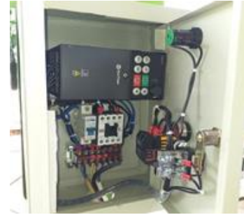
Figure 4b. Gear box added inverter
