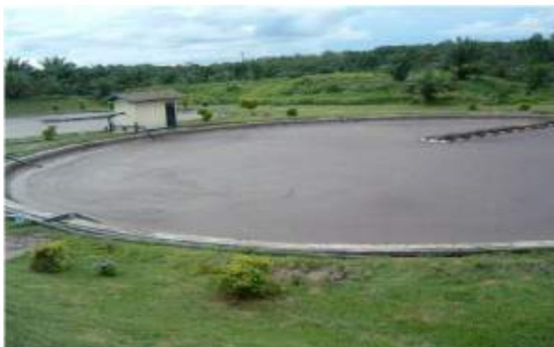
Figure 34.11. Open anaerobic pond for POME treatment
