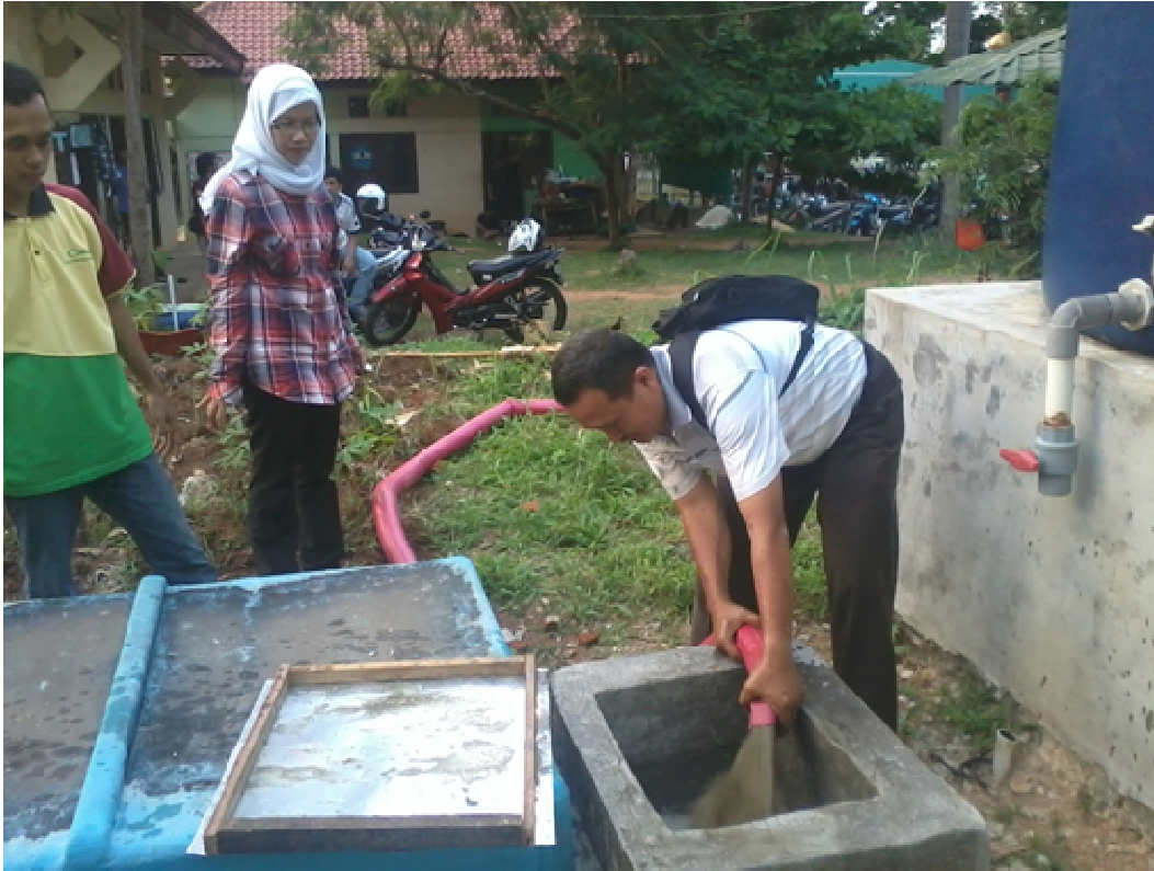
Gambar 12. Pengisian bak digester
