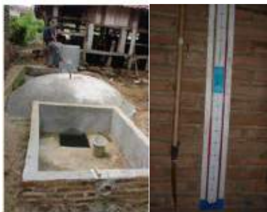
Figure 1. Fixed dome biogas digester and simple water manometer.
