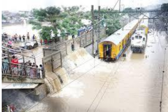
Figure 2. Overtopping and failure of flood defences ( The Jakarta Post, 2013)
