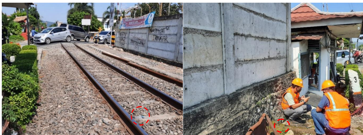
Figure 3. Accelerometer sensors was located at sleeper on left picture and another one on the ground.
