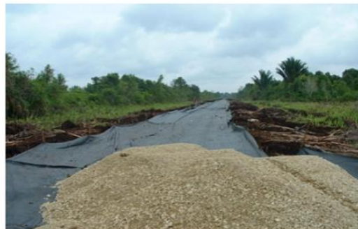
Figure 11: Application of Woven Geotextiles (woven)
