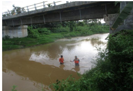
Figure 5. Discharge measurement at Giri Tunggal Bridge, Way Wayah River
