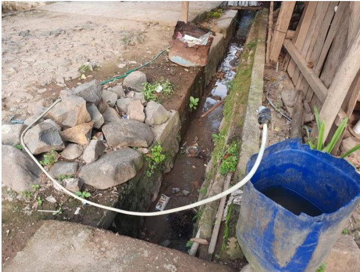
Picture 30. PAMSIMAS piping
