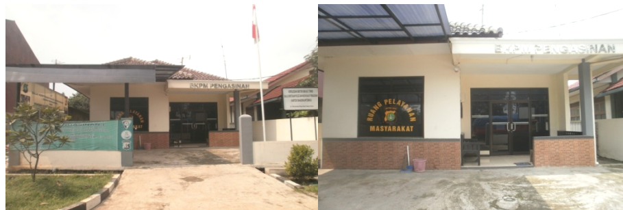
Photo 8. Front and Close Up of BKPM Pengasinan
