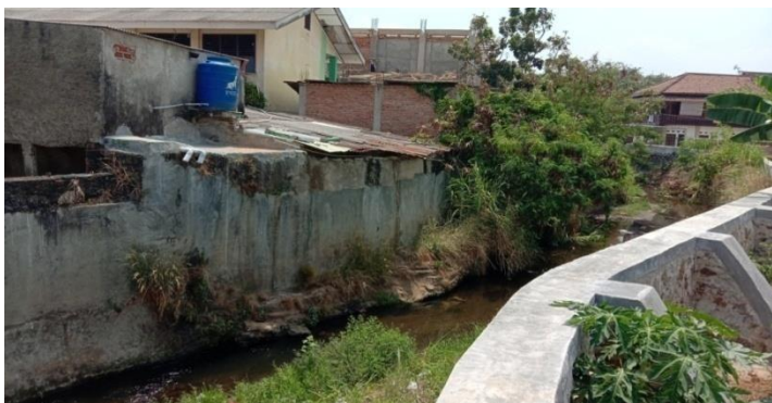
Figure 2. Situation at riverbank of Way Balau River.
