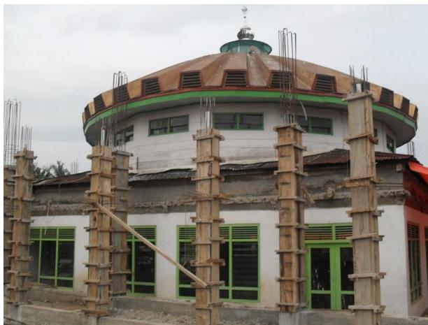
Figure 1. Roof dome of Hidayatullah Mosque was made of aluminum zink at construction stage before removed.
