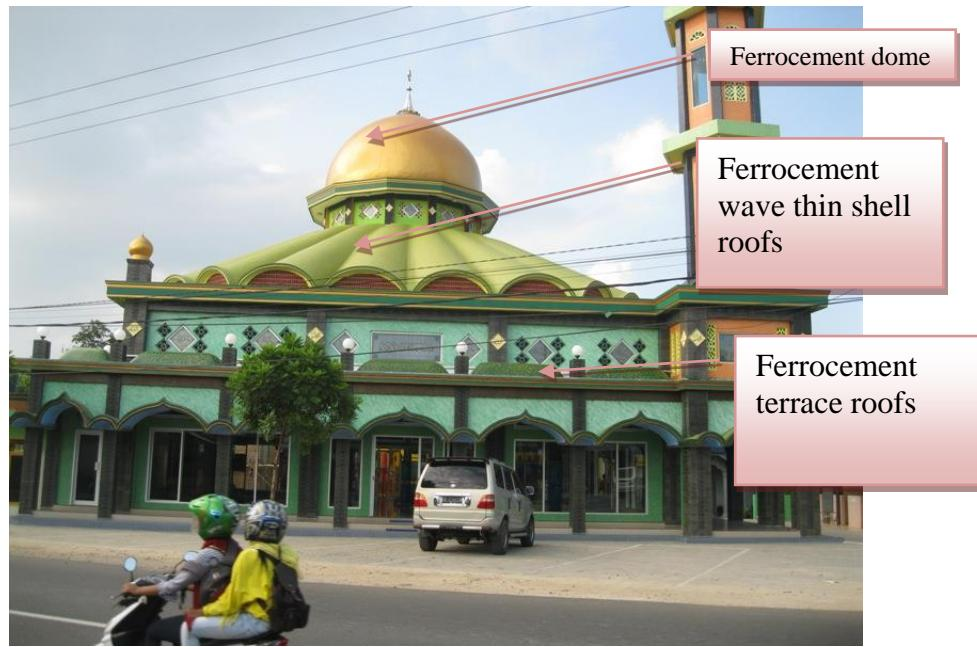
Figure 3. Ferrocement Structure on Dome, main roofs and terrace roofs.
