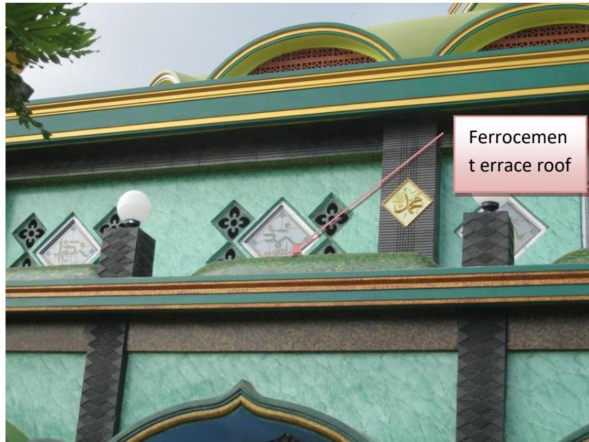
Figure 7. Appication of ferrocement on terrace roofs from outside.
