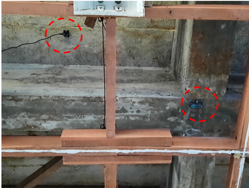
Figure 4. Two accelerometer for recording acceleration of slab and beam.
