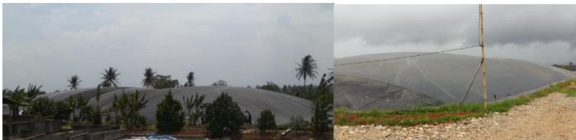
Figure 2. Covered lagoon biogas digester facility in PD. Semangat Jaya at different times and views.
