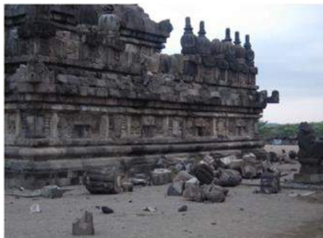
Figure 2. Damage of Prambanan Temple due to the 2006 Yogyakarta earthquake [3]
