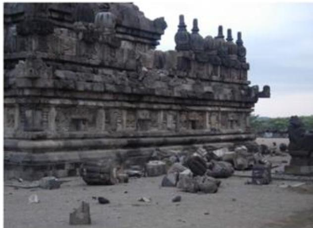
Figure 2. Damage of Prambanan Temple due to the 2006 Yogyakarta earthquake<sup>[3]</sup>
