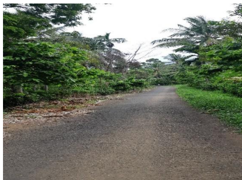
Gambar 4. Kondisi jalan menuju KLS Figure 4. Road condition to KLS
