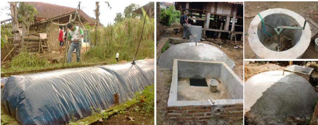
Figure 2. (a) Tubular plastic digester, and (b) fixed dome concrete digester.
