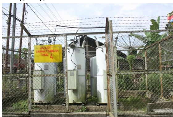
Gbr. 1. Step Voltage Regulator
