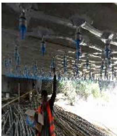
Figure 4. Cracks repairing process.
