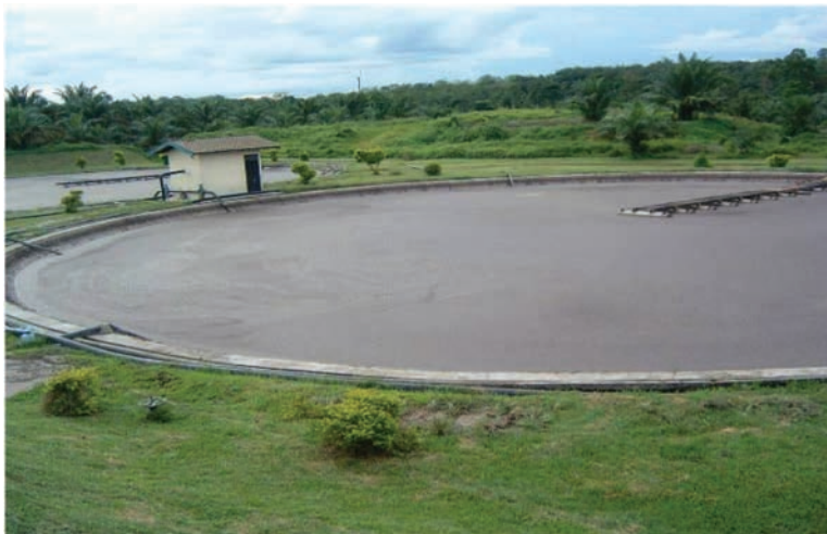
Figure 27.9. Open anaerobic pond for POME treatment
