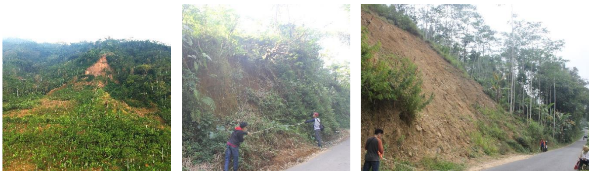
Figure 4. Landslides in Karangkoobar Catchment
