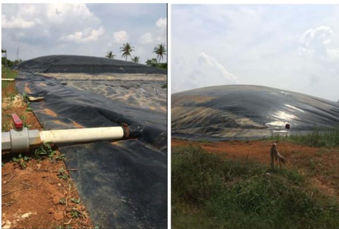
Figure 2. Biogas digester at PD. Semangat Jaya
