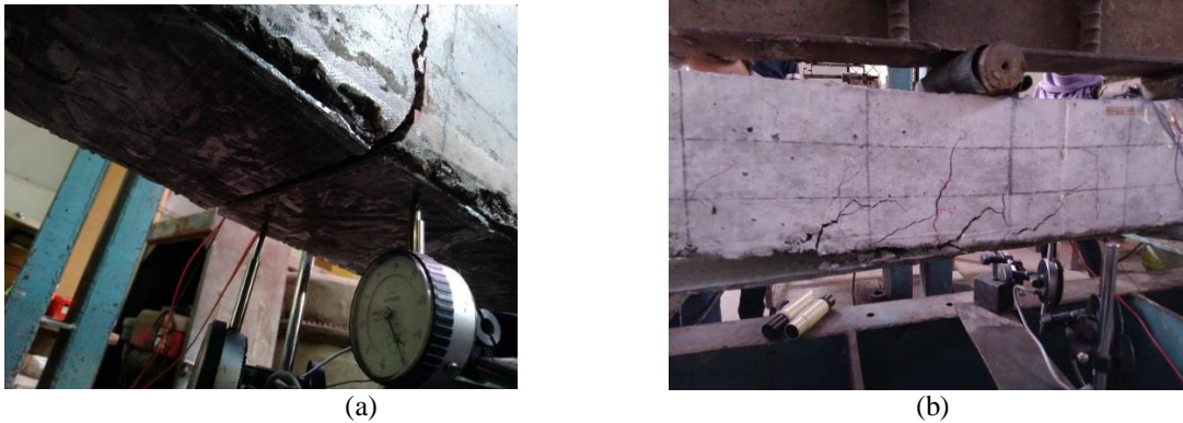
Figure 8. (a) Strengthening beam (B2) failed due to laminate snap at mid-span bottom beam; (b) Beam B3 failed due to de-bonding at one end laminated.
